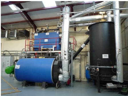
Figure 8.34. Cogeneration station with gasification factor, gas boiler and 35 kW power Stirling engine (Photos Ů. Kask)
