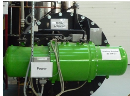
Figure 8.34. Cogeneration station with gasification factor, gas boiler and 35 kW power Stirling engine (Photos Ů. Kask)
