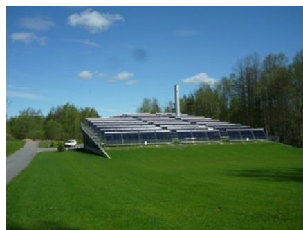
Figure 8.5. Installation of solar panels at the Pühajärve wood-fired district heating boiler house. (Photo Ü. Kask)
